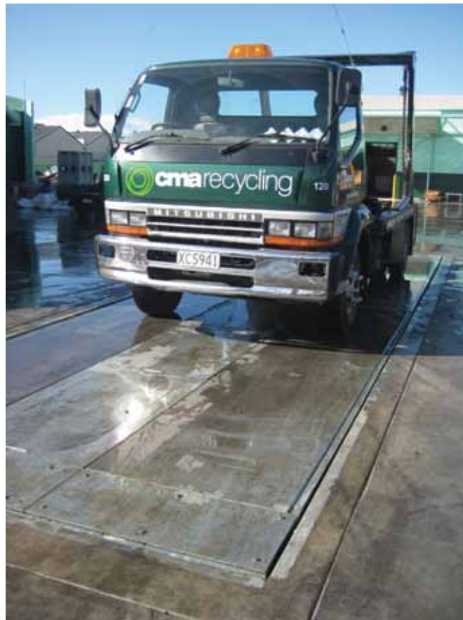
FULLY IN-GROUND INSTALLATION
