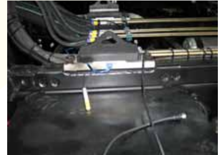
SWEDISH 13" LOADCELL INSTALLED
